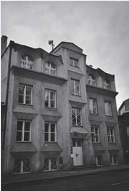
Cubist house in Prague
