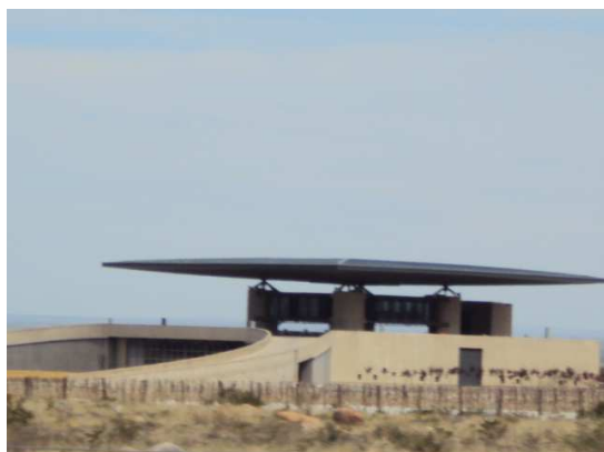
Vista exterior Bodega O' Fournier.
